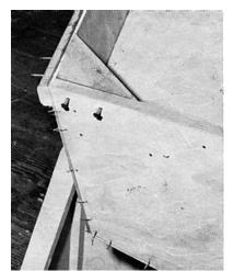
These are two triangular pieces of hardwood that fit into the top aft corners of the boat to strengthen the structure.
