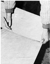
Draw a vertical line exactly down the centre on both sides of the **aft transom (7)**. Use these lines to match the transom with the seam of the bottom panels. Mark off corresponding lace holes on the lower edge of the transom against the corresponding holes in the after edge of the bottom panel –  $\frac{1}{4}$  " (6 mm) from the edge.
