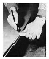
Place the one bottom section on top of the other, with butt straps on the inside, so that the two shapes match exactly and the cutaway portions that will form the centrecase slot are together. Draw a pencil line  $\frac{1}{4}$ " (6 mm) from
